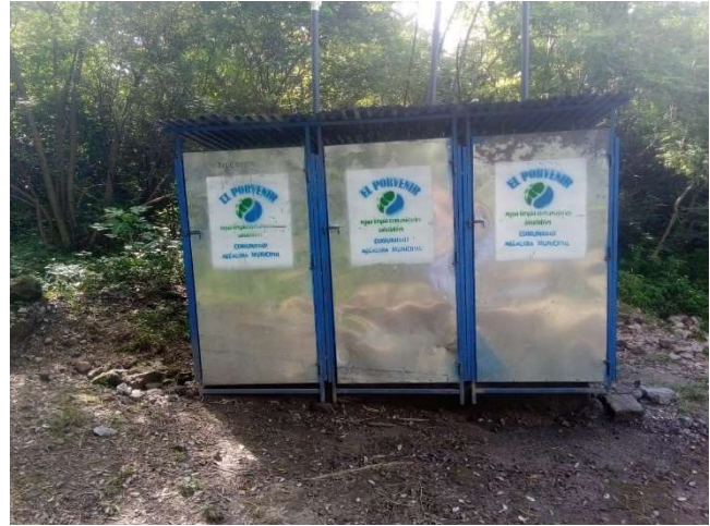
Because there are so few students (15), the latrine pits will not fill up as fast. Therefore simple, single-pit latrines were built in Playa de Moyua.
